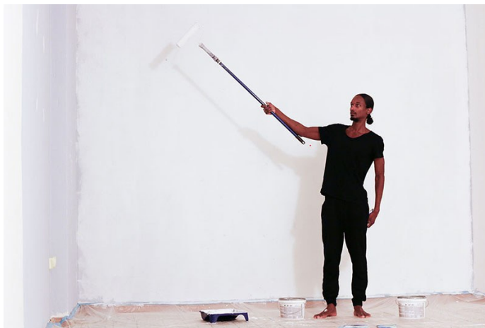
Figure 5: A painter uses an extension roller to paint a wall.
